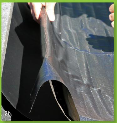
a. Place the ND Drainage Systems with the flange side (strip without dimples) and the not-flange side against each other.
